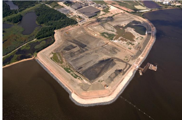
The Cox Creek Dredged Material Containment Facility is an important placement site for material dredged from the Baltimore Harbor.
