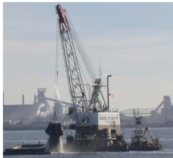
A mechanical dredge in the Baltimore Harbor.
