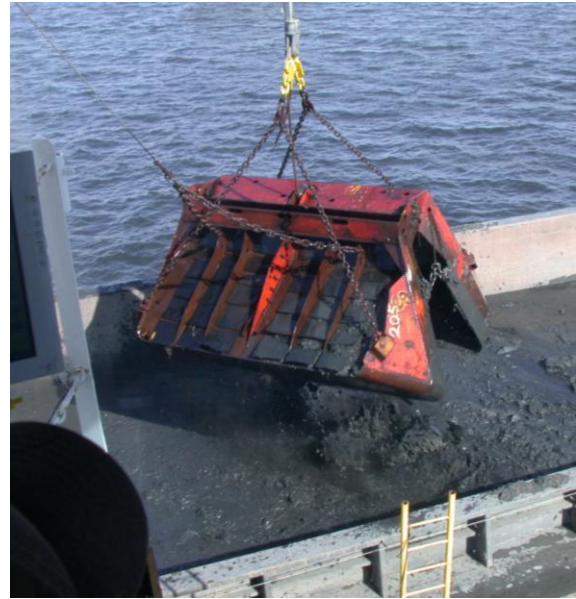
A clamshell bucket depositing dredged material onto a barge.
