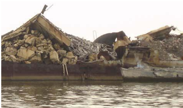
Before the clean-up, piles of waste from past industrial activity dominated the scene at Masonville.
